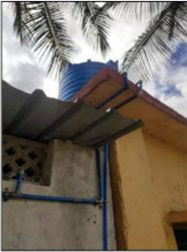
Fig-1: Nelwy installed over-head tank
