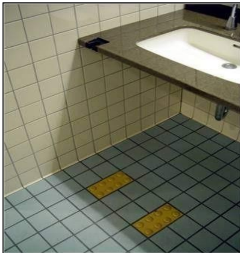
Figure 5.27 Warning pavers
